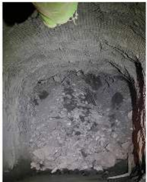
Figure 4 Drilling the first stope (LHS) and drawpoint after firing
